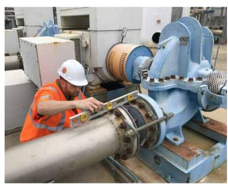
IMAGE 1: User conducting an expansion joint survey (Images courtesy of Proco Products)
