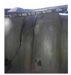
IMAGE 3: Inspect expansion joints for abnormal wear to help catch problems before they happen
