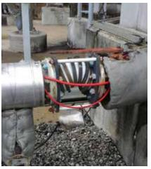
IMAGE 2: Faulty expansion joint installation
