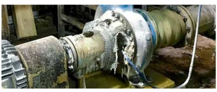
IMAGE 1: A damaged shaft leads to reduced sealing quality (Image courtesy of FSA)
