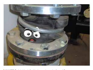
IMAGE 3: Joint installed between two misaligned flanges.
