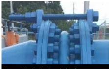
Image 6. Locked out control rod
