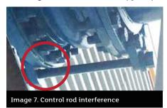
be found on expansion joints with excessive lateral offset, tapered reducing joints or a control unit assembly not specified to the correct application.
