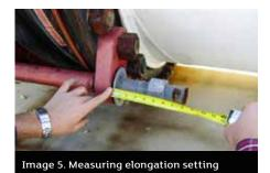
Control units can be adjusted at any time, and it is not too late to make corrections in the field. In addition to adjustments made to the nuts, the gusset plate along with the entire rod assembly can be relocated for better spacing without breaking the seal between the rubber joint and pipe flange.
